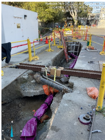
6" RW pipeline at WWTF
