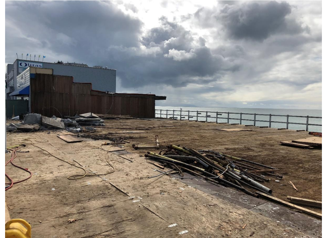
PILING REPLACEMENT PROJECT (Miramar Demo)
