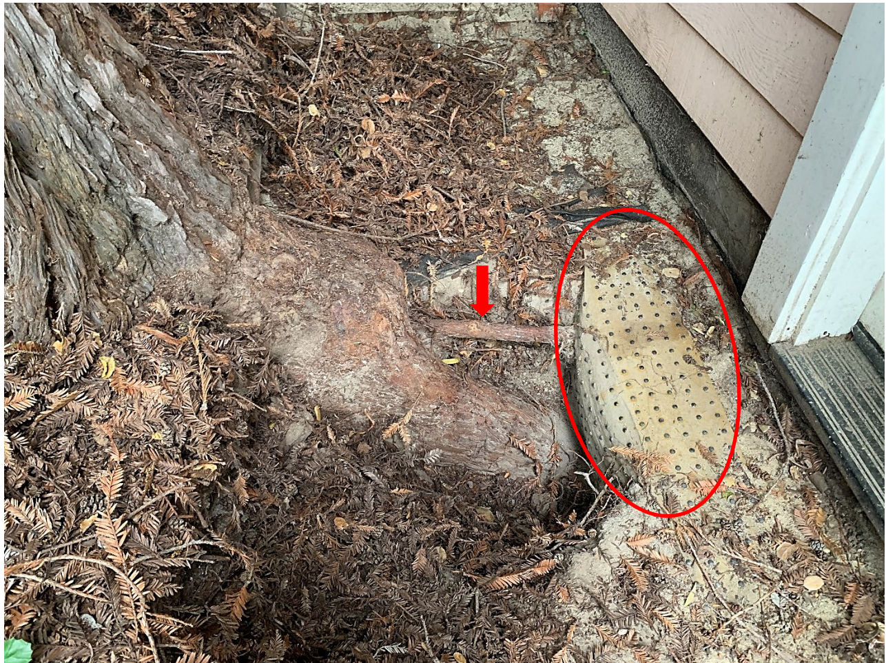
Image #6 – Tree T2, redwood and 8” diameter buttress root. Note root is growing below root barrier. Second 2” root arrow.
