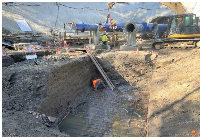
Photo 9: Newell Creek Dam Inlet/Outlet Replacement – Installation of Rebar for Outlet Structure
