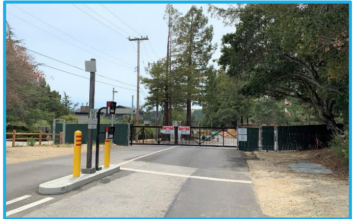
Photo 19: GHWTP Entrance Improvements - New Entry Gates in the Closed Position and Access Pad from the Outside
