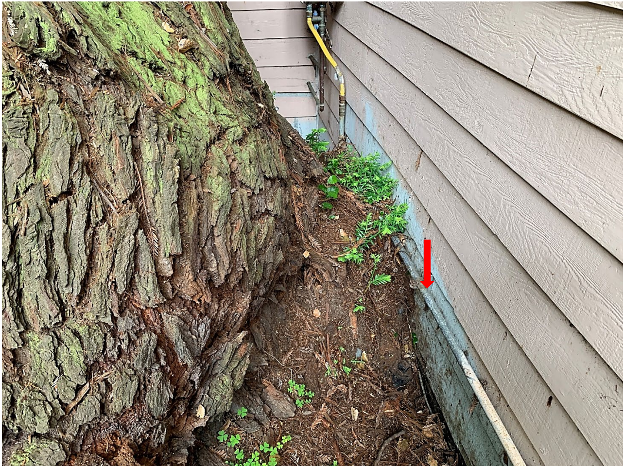
Image #2 –Tree T1, coast redwood. Note trunk growing against home siding. Also note trunk is very close to gas line running against home siding, (arrow).
