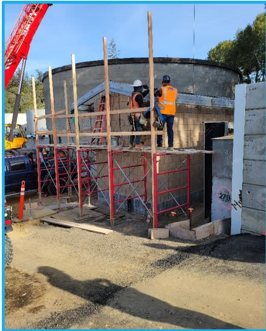
Photo 11: GHWTP Concrete Tanks Replacement – Framing Roof of New Electrical Building
