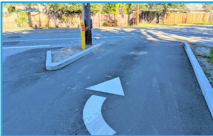
Photo 20: GHWTP Entrance Improvements - New Right Exit Lane with Newly Striped Bollard
