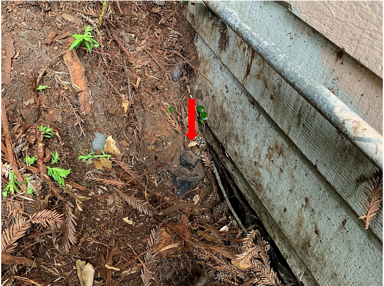
Image #4 –Tree T1, note sewer clean out. (arrow).
