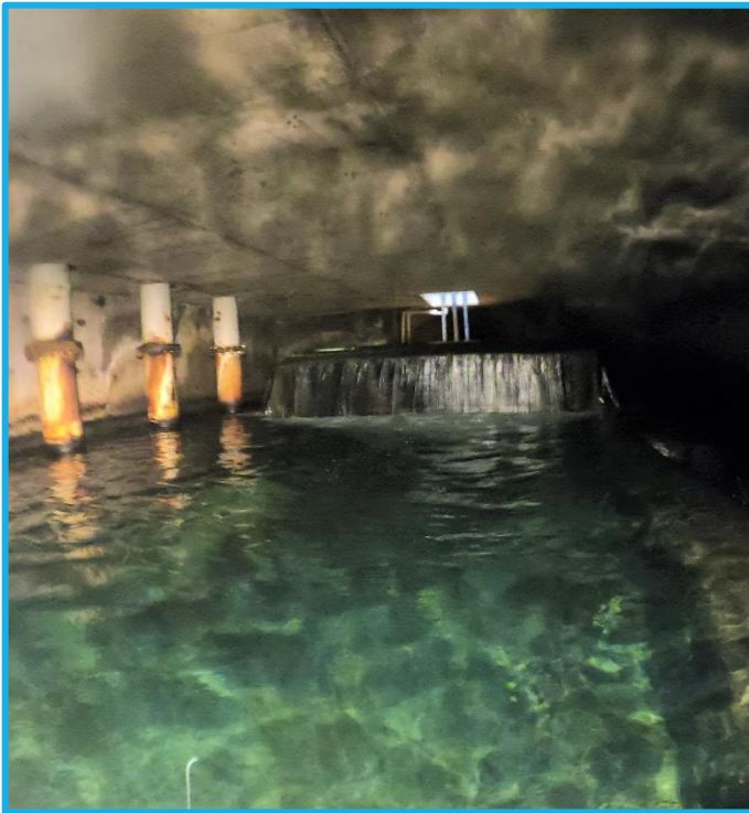
Photo 1: GHTWP Facility Improvements - Clearwell Inspection
