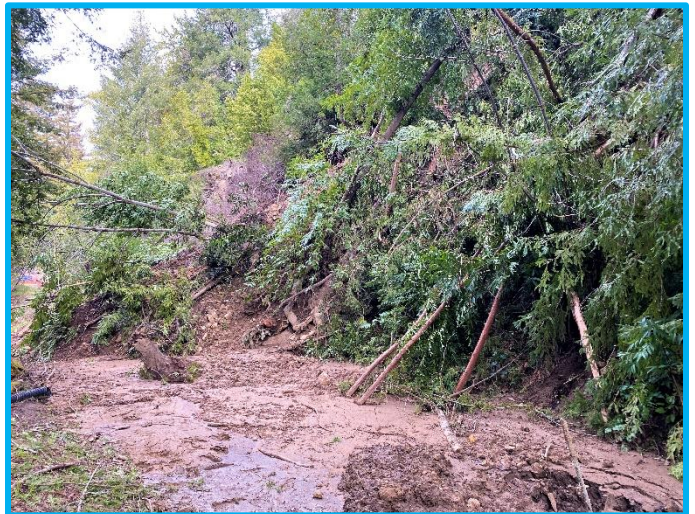
Photo 4: Brackney Landslide Area after Winter Storms
