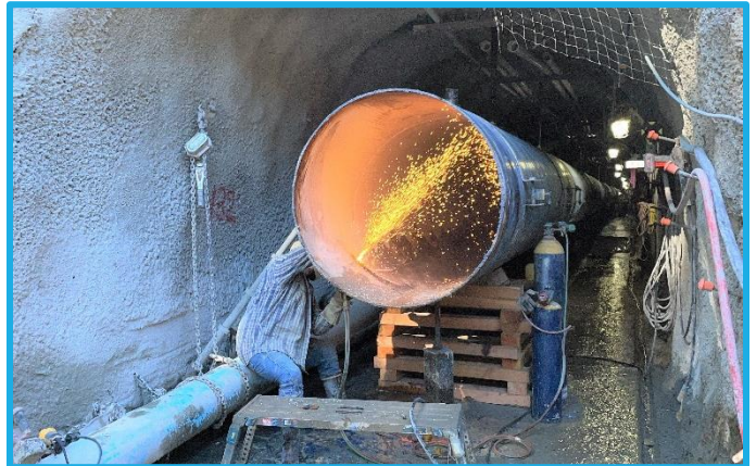
Photo 8: Newell Creek Dam Inlet/Outlet Replacement – Welding on 48" Steel Pipe at Sta 11+00
