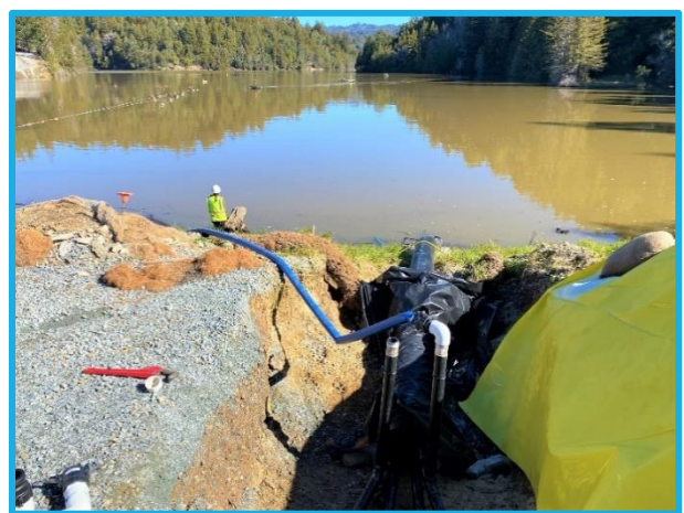
Photo 10: Newell Creek Dam Inlet/Outlet Replacement – LOX System Startup
