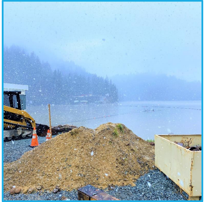
Photo 6: Newell Creek Dam Inlet/Outlet Replacement – Snow Fall
