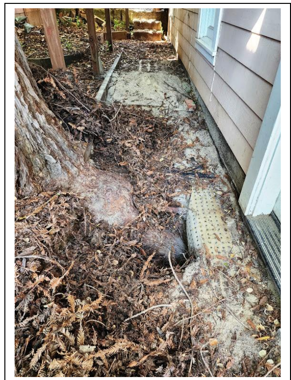
Root flare expansion with large structural root encroaching under foundation.
