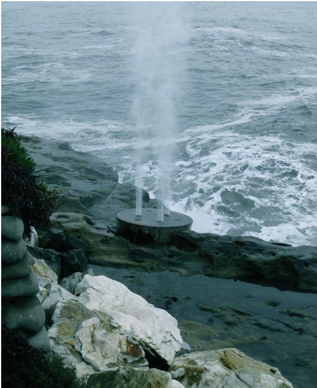
Figure 3-13. Concrete cork-like cap over former wave motor shaft was fitted with three PVC pipes to relieve pressure from wave surge and now serves as a natural blowhole.
