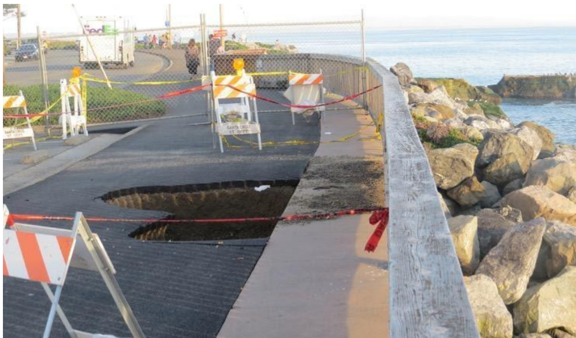
Figure 3-9. Collapse of one of the parking areas along West Cliff due to wave undermining of a seawall just west of Columbia Street followed by collapse of overlying fill material (Zone 2).
