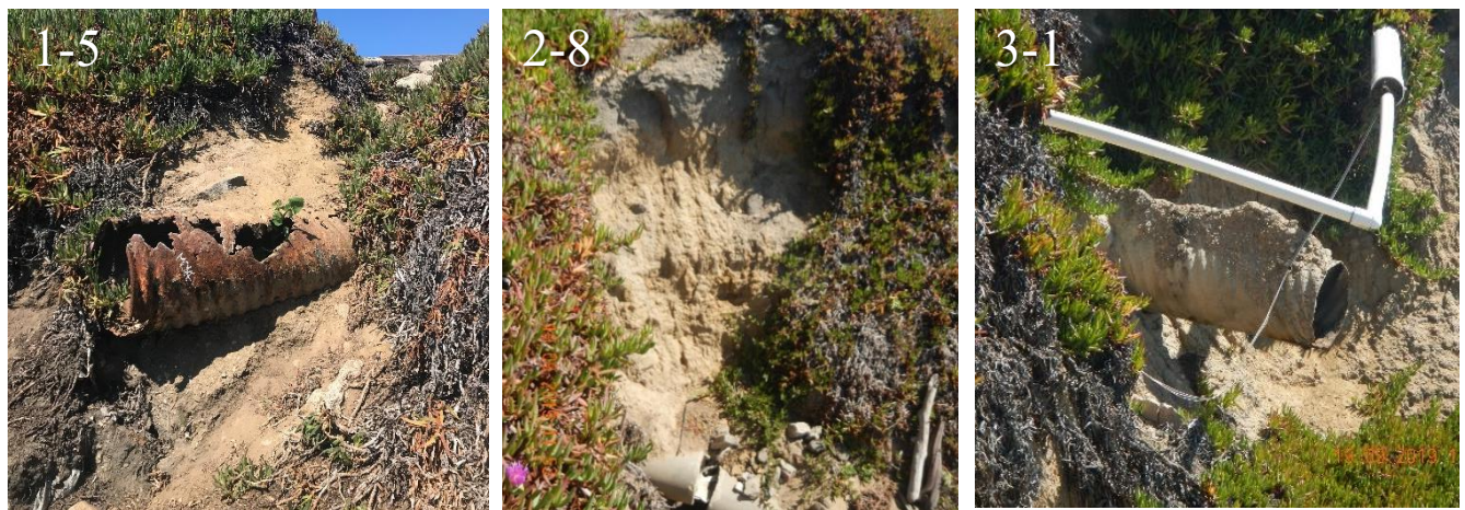
Figure 4-2. Examples of failing stormwater infrastructure
