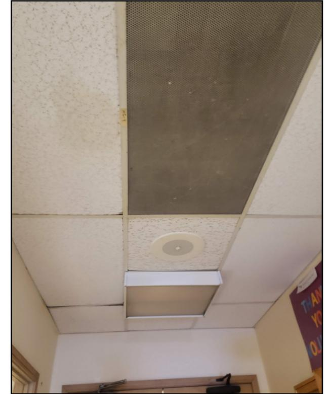
*Deteriorating and water damaged ceilings*
