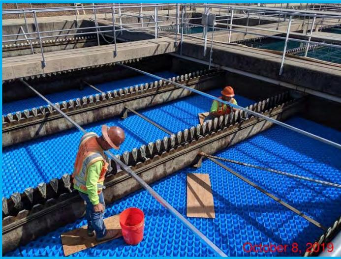
**Figure 9 – GHWTP Tube Settler Installation**
